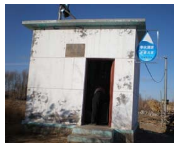
Water pumping station
